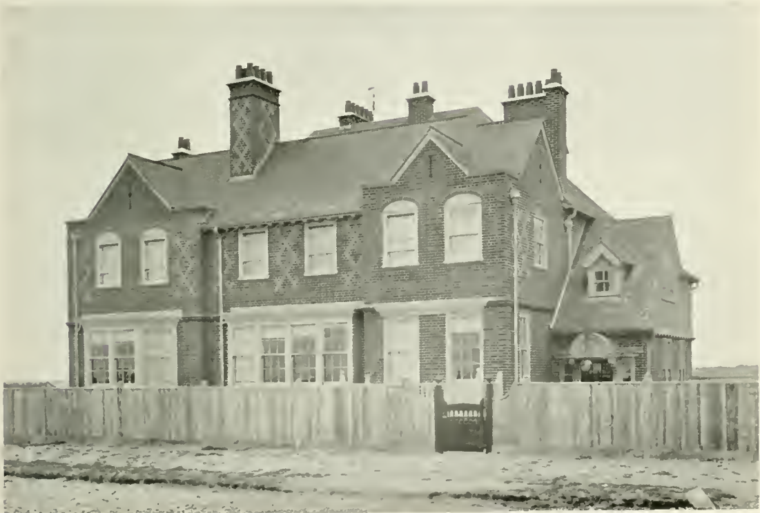
B46 SANDYCROFT, LITTLESTONE-ON-SEA, BUILT FOR THE RIGHT HON. HERBERT J. GLADSTONE, M.P. MATERIALS, DARK RED BRICK FACINGS, BROWN TILE ROOF, THE WINDOW FRAMES AND THE WOODWORK PAINTED WHITE.
